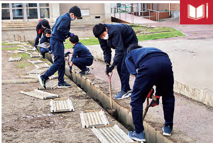
Raising ground gutters
